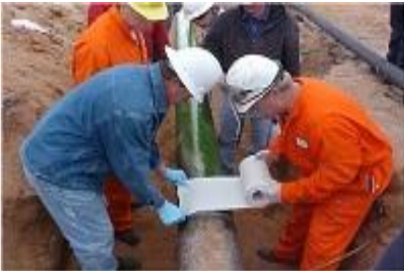
Wet-layup ready to apply right out of the bag, requires no field-mixing of cloth with epoxy resin minutes prior to install.
