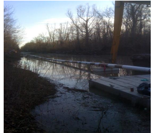
Many isolated external corrosion >80% reinforced. Water nor sweating lines causes any issues!
