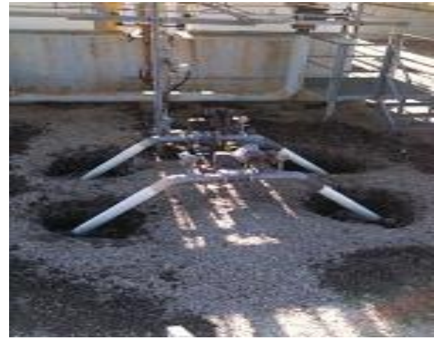
Soil to air interface repair in one hour , 2"x10'
