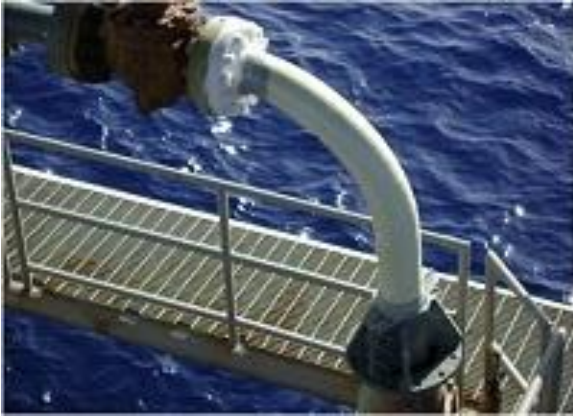
Elbow repaired with composite in less than one hour
