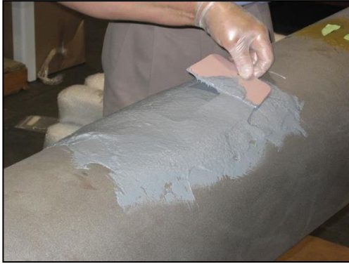
Fig. 3 – The defect must be completely filled in and the compound must be smoothed and leveled out. Remove high spots and fill any low spots
