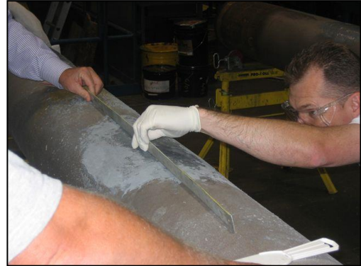
Fig. 4 – Use a straight edge to confirm evenness.
